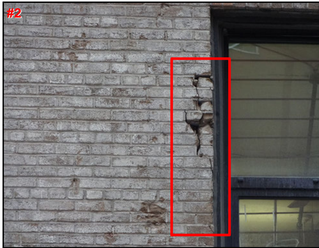
Missing and damaged brickwork.
