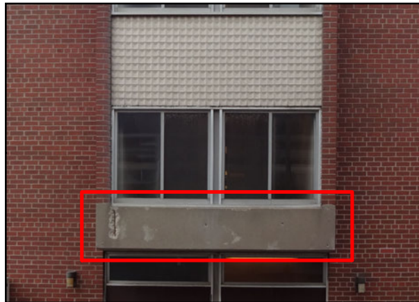
#4: Concrete spalling
