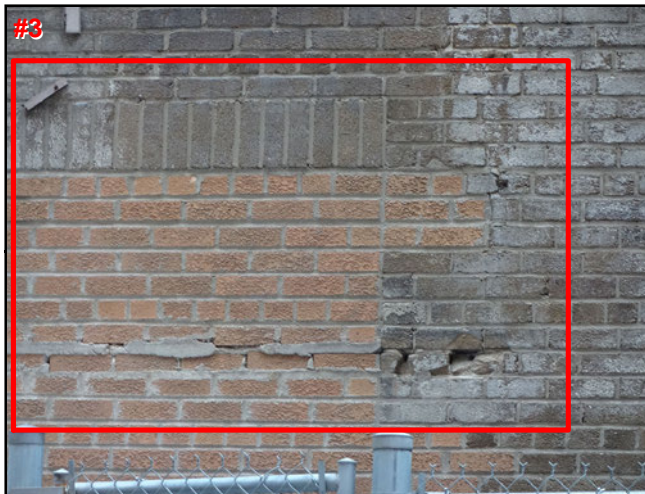
Deficiency in wall fabric increases deterioration of mortar and brick, and promotes water entry.
