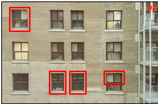
Suspect heat loss from windows.
